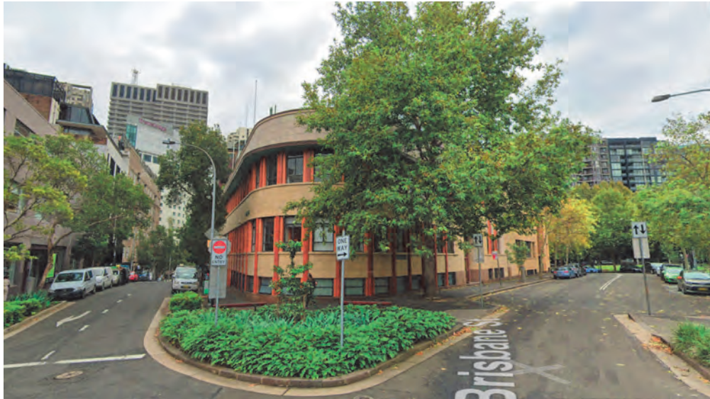
Figure 1: Photo from Hunt Street
