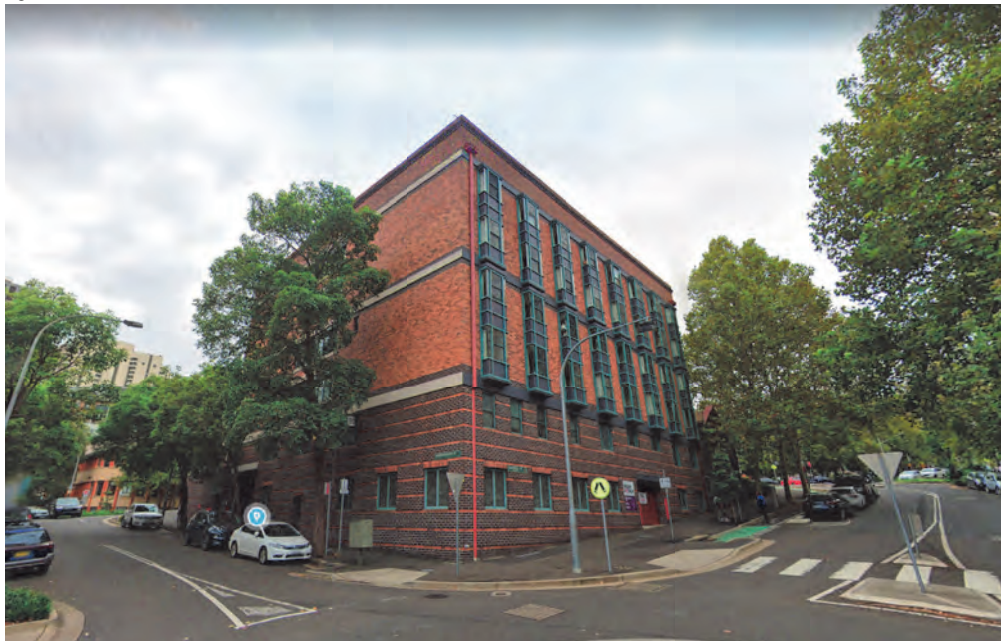
Figure 2: Photo from Hunt Street
