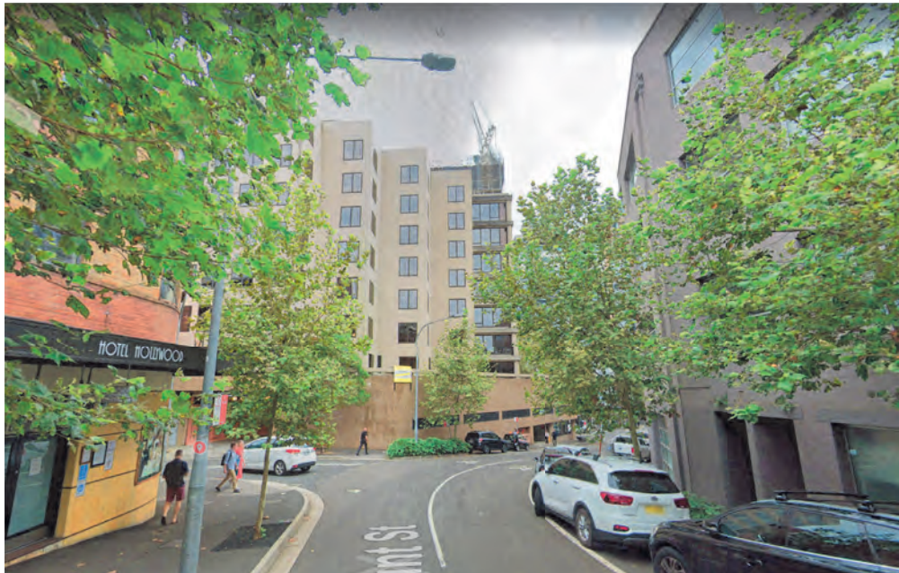
Figure 2: Photo from Hunt Street
