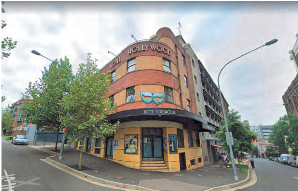
Figure 2: Photo from Hunt Street
